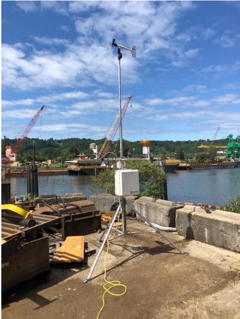
Figure 2. Site 1 Monitoring System
