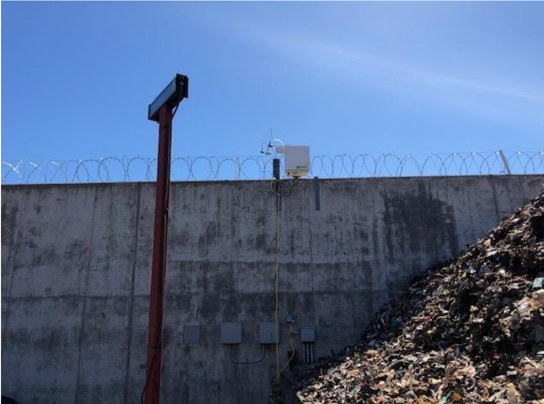
Figure 5. Site 4 Monitoring System
